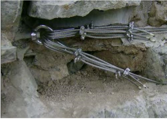
Detail of the anchoring system of the strands
