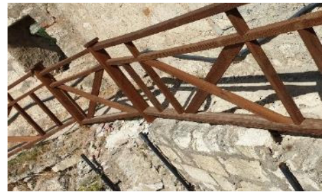
A child can fall through the mesh of the railing
