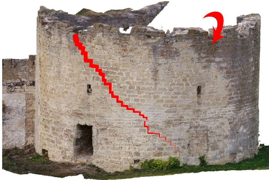
Typical kinematical motion of a portion of masonry in case of circular buildings such as Tower B3
